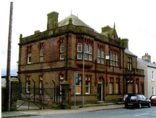
Original Frizington Council Headquarters
