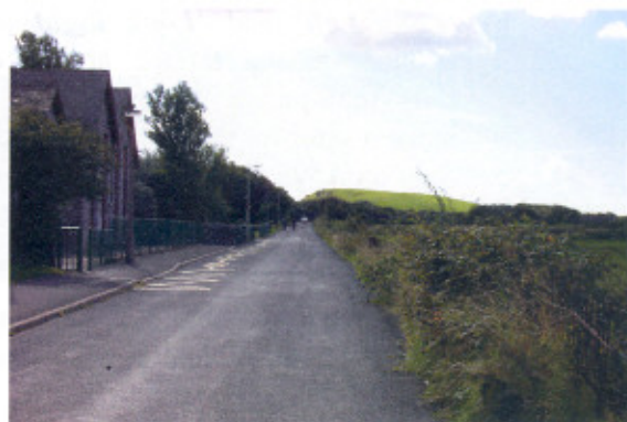
Lots Road outside Askam Village School. On a busy school day this road can be very easily blocked. The widening of the road and provision of a footway should increase safe walking to school.
