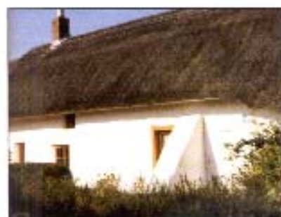
LONGBURGH HALL A GOOD EXAMPLE OF WATTLE DAUB CONSTRUCTION
