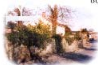
COBBLED WALL RUNS INTERMITTENTLY THROUGHOUT THE LENGTH OF THE VILLAGE
